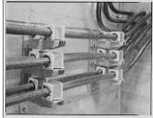
12 kV Service Duct Bank
